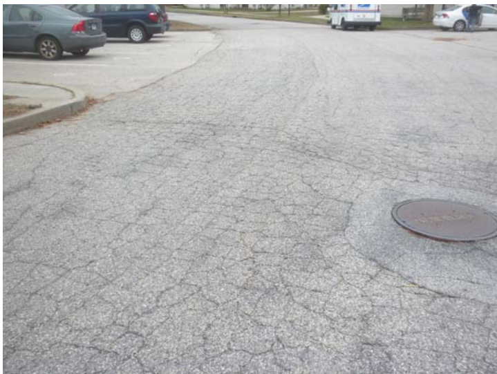
Cracking original asphalt
