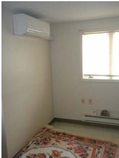
Recently install split system heat pump unit register
