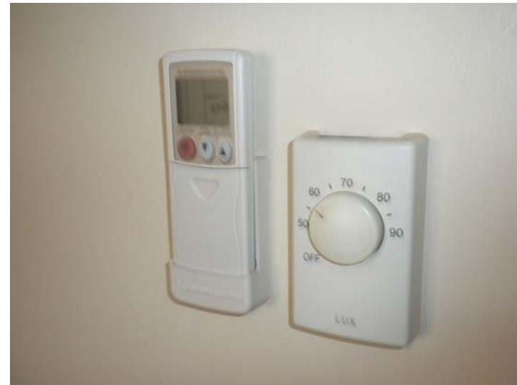
"Newer" thermostat control and heat pump control
