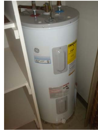
Unit electric domestic hot water tank
